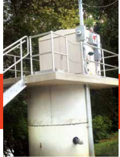
The city of Marietta's engineering department designed the facility upgrade.
