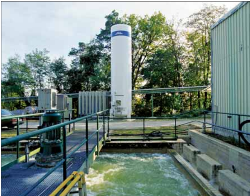
Linde gas diffusion water treatment pond
