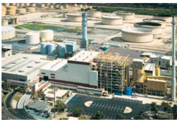
Plant view facing north
