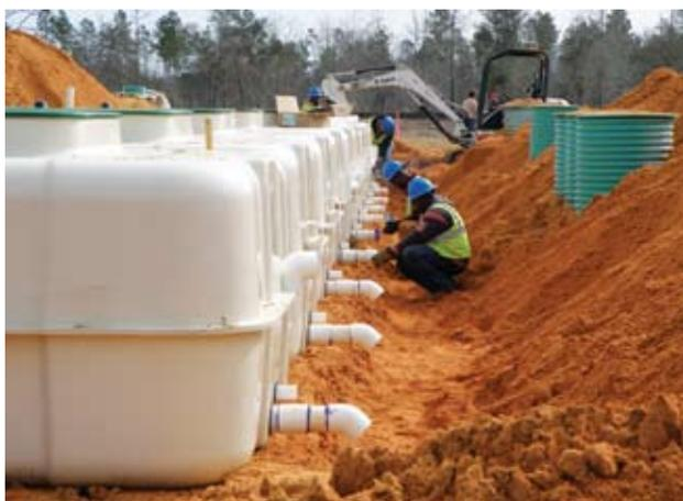
The AeroCell system is a pre-engineered synthetic media filter utilizing open-cell foam cubes housed inside individual fiberglass enclosures. Open-cell foam has been proven over the past 15 years to treat wastewater to secondary or better levels.
